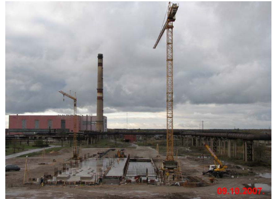
Foundation of UTT-3000 on Viru Keemia Group Galoter Project Site in Kohtla Yarve, Estonia, made under ATOMENERGOPROEKT's design, 9 th Oct, 2007
